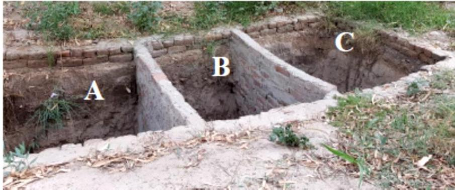
Fig. 2: Pits for solid waste management.
