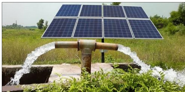
Fig. 3: Groundwater extraction with the use of solar power (original field photograph taken by the authors during the 2023 survey). Source: Field survey, 2023.
